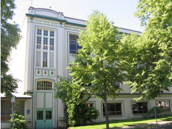
North elevation facing south
