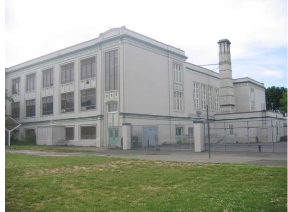
South elevation facing northeast
