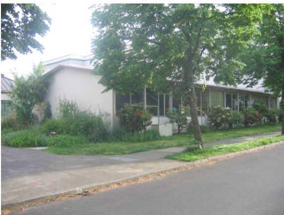
North and east elevation 1960 addition
